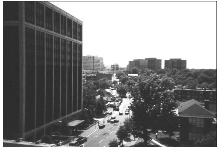
WRIT PROJECT. 1600 Wilson Boulevard and the 7-11 are included in the assemblage of properties that will include two new apartment buildings.
